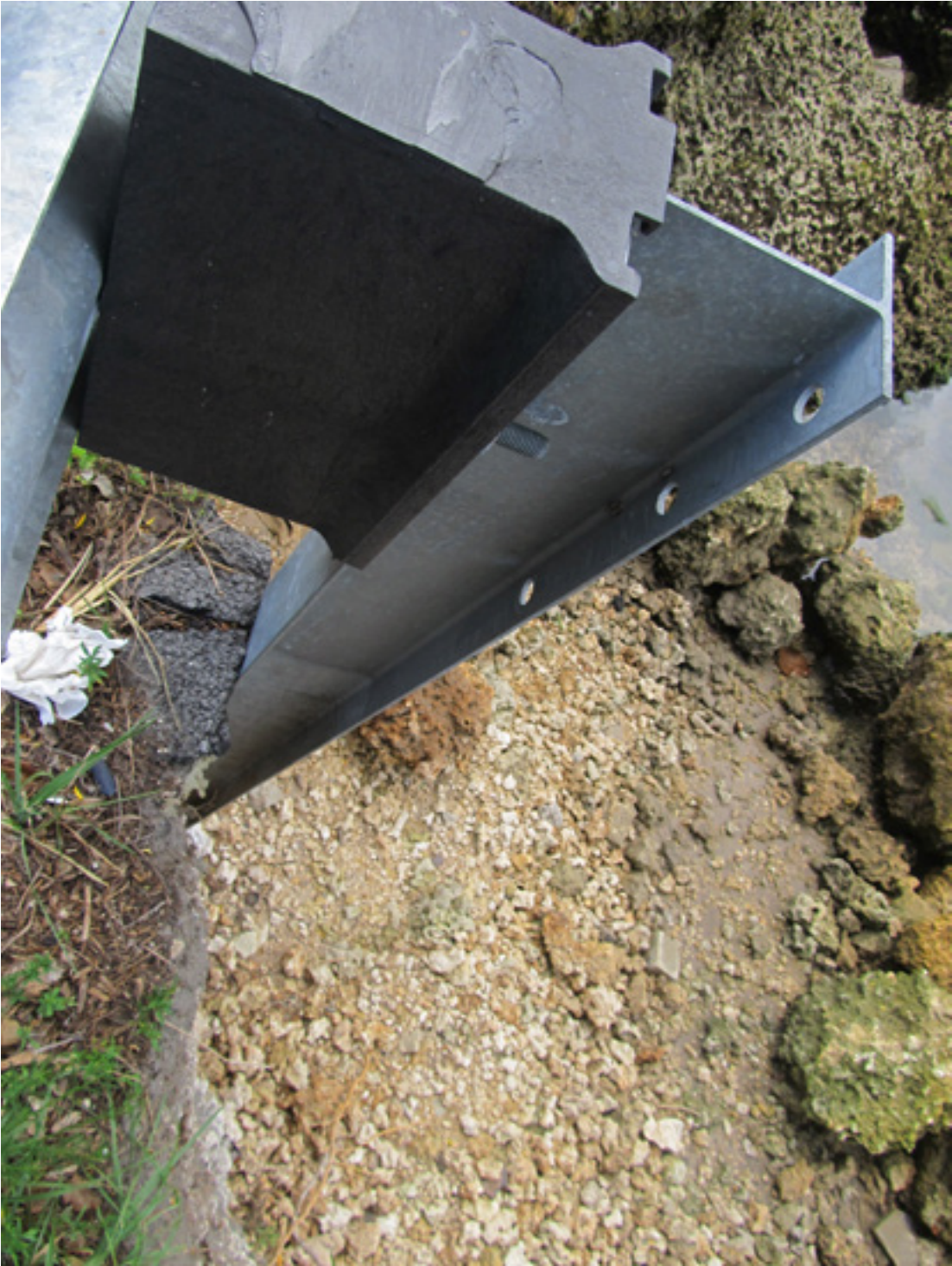
On Road Greenway 2810 NW South River Dr.
