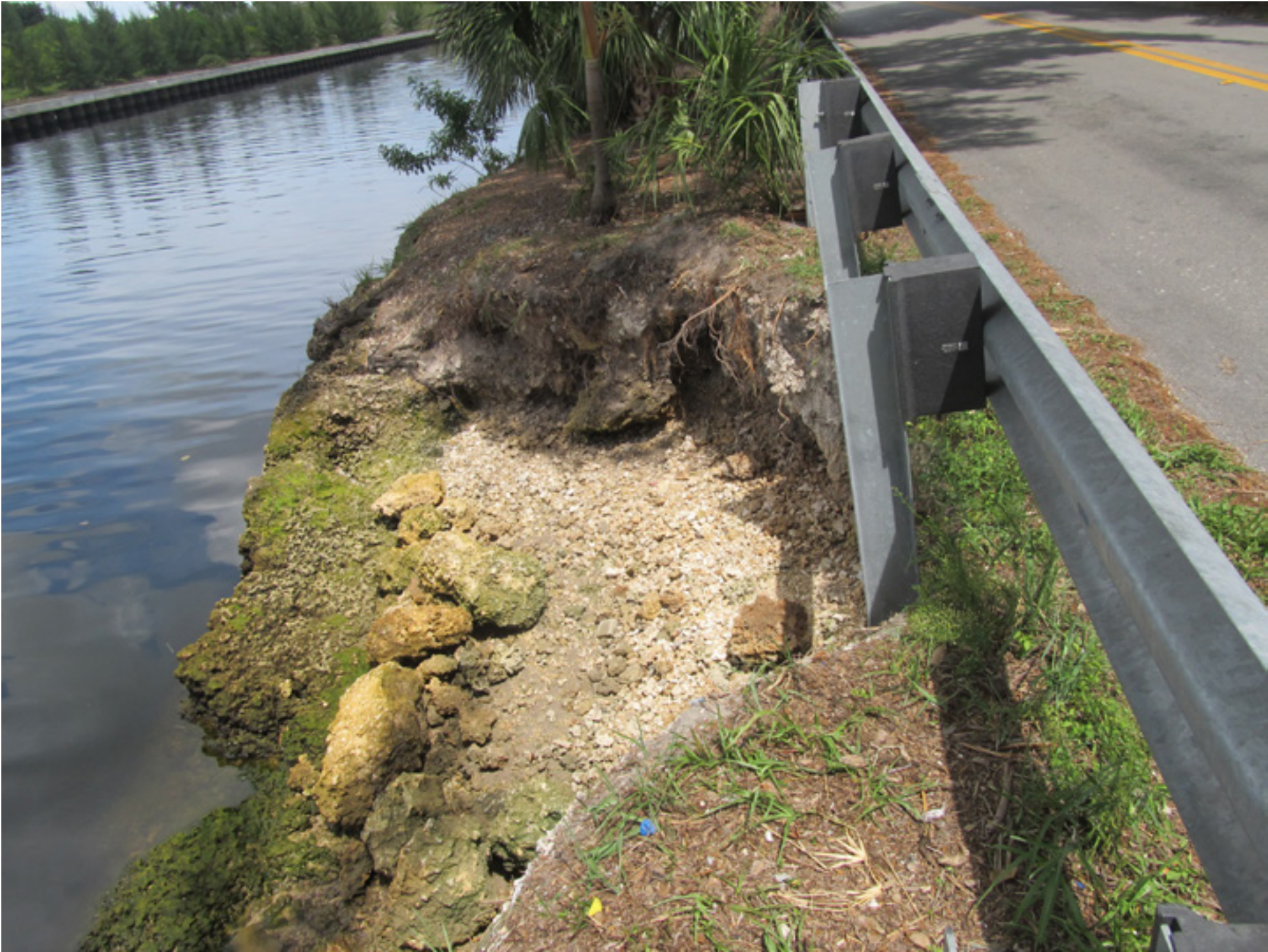
On Road Greenway 2810 NW South River Dr.
