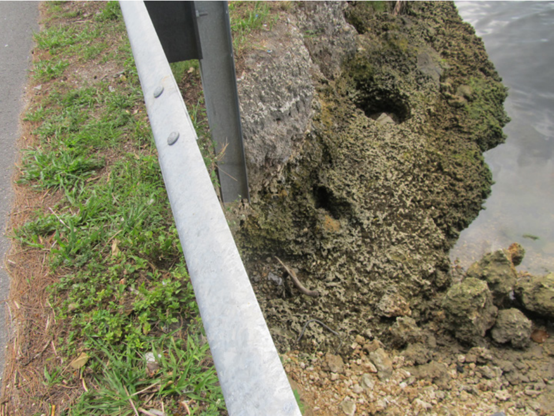
On Road Greenway 2810 NW South River Dr.
