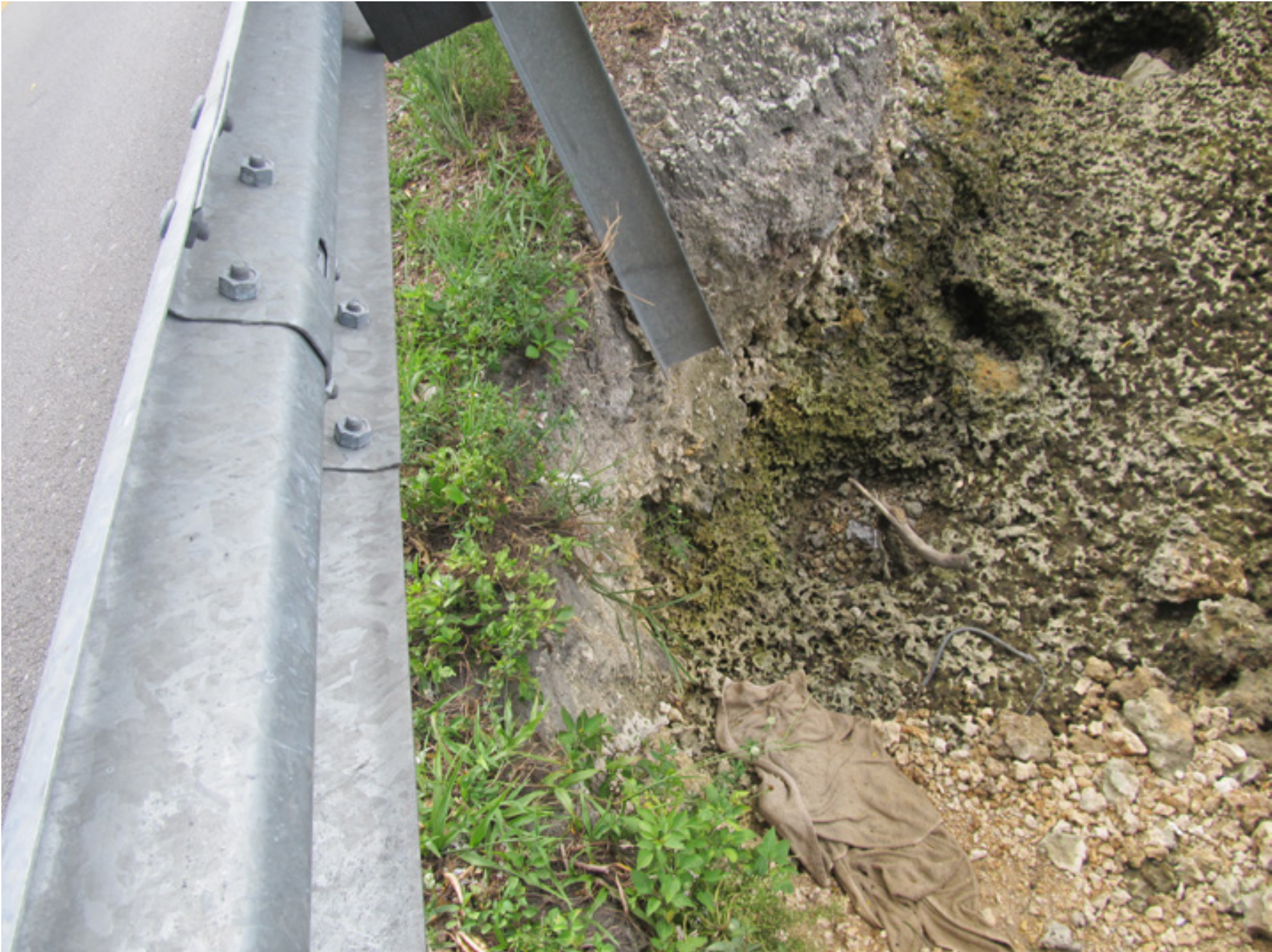
On Road Greenway 2810 NW South River Dr.
